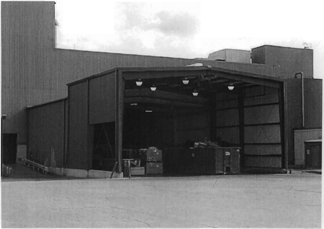
9. South Waste Compactor Area under roof and secondary containment.
