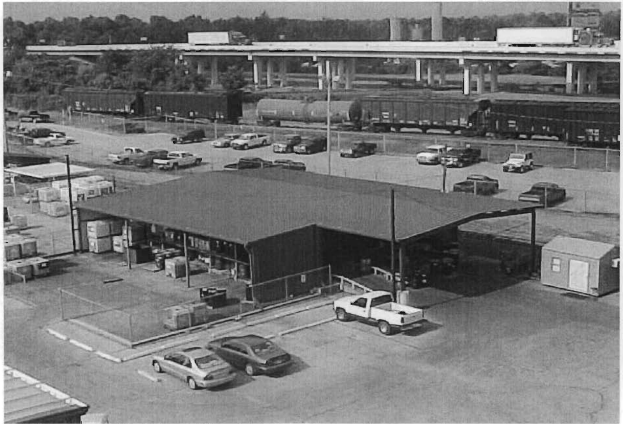
2. Oil Storage Area after BMPs. Additional cover over containers, all containers within secondary containment.
