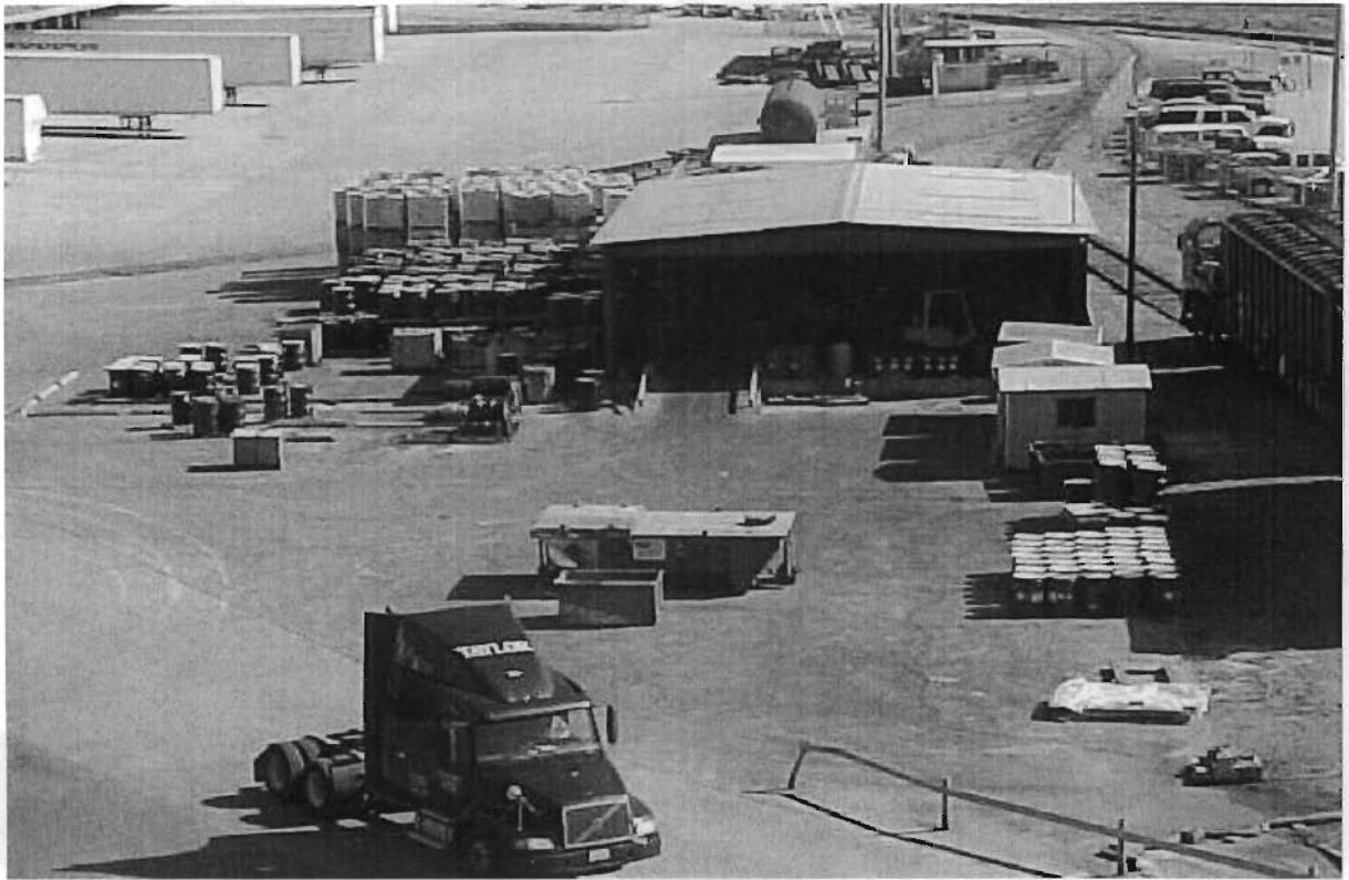
1. Oil Storage Area prior to BMPs. Containers exposed to stormwater.
