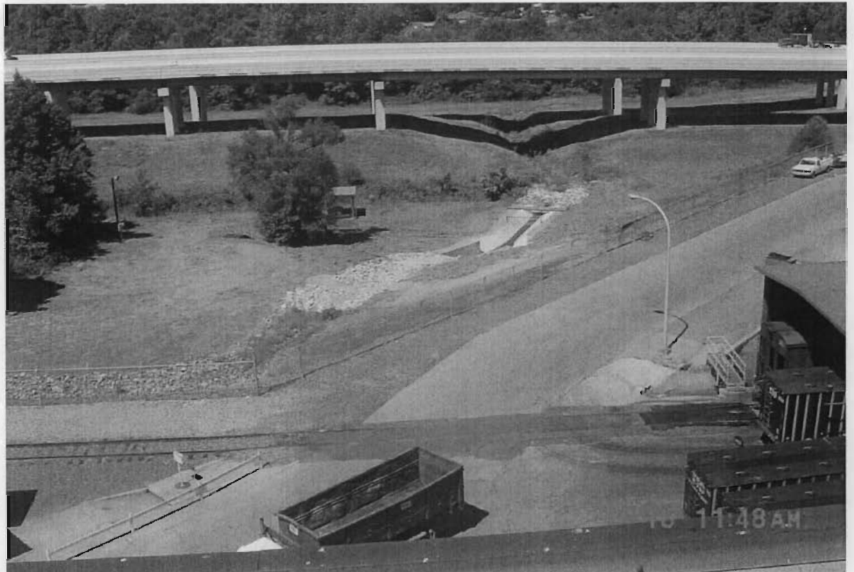
17. Outfall 001 after BMPs.
