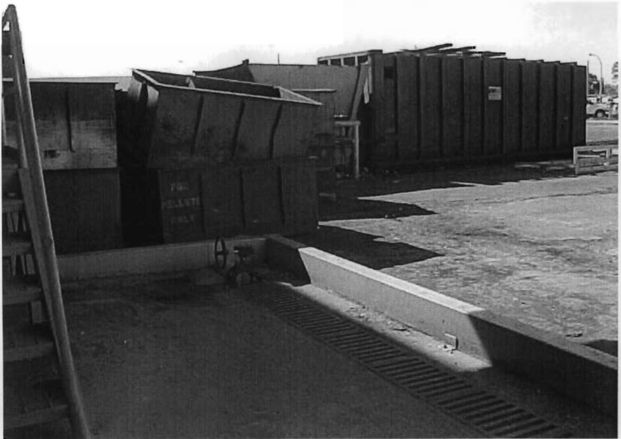
10. North Waste Compactor Area before BMPs. Potential exposure to stormwater.
