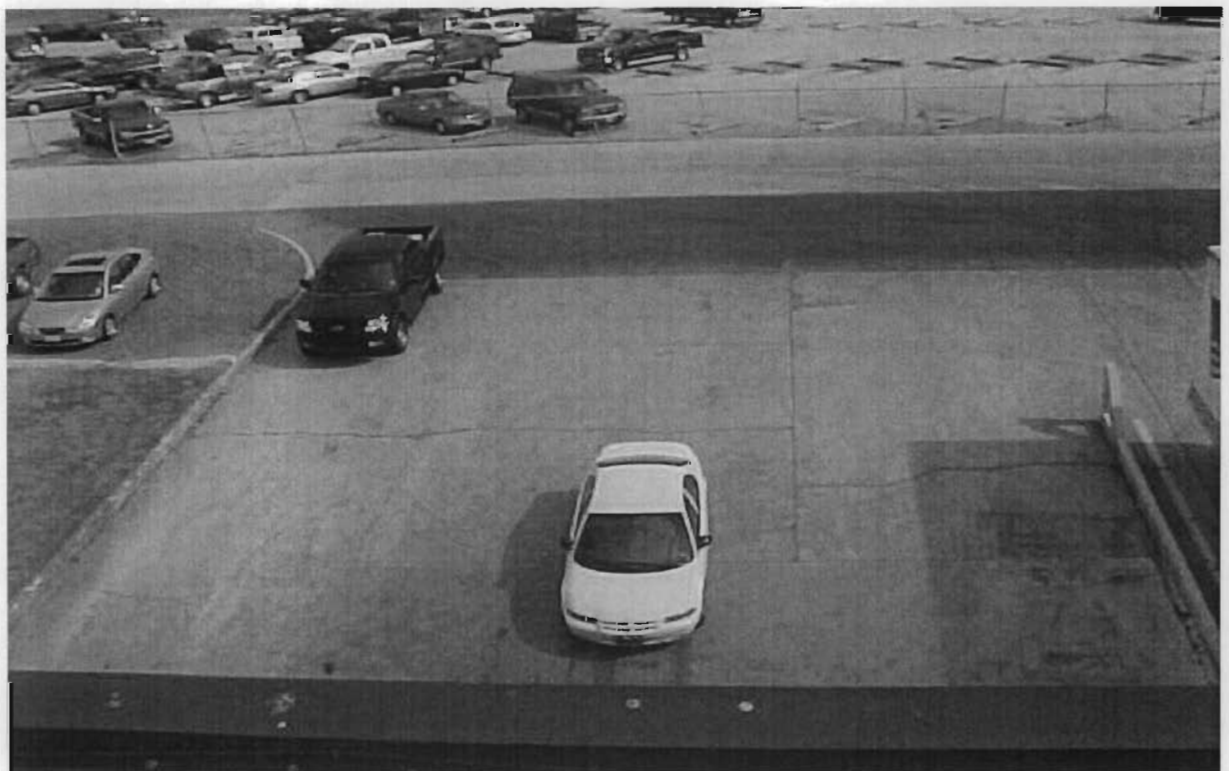
11. North Waste Compactor Area after BMPs. Relocated under cover to South Compactor Area.
