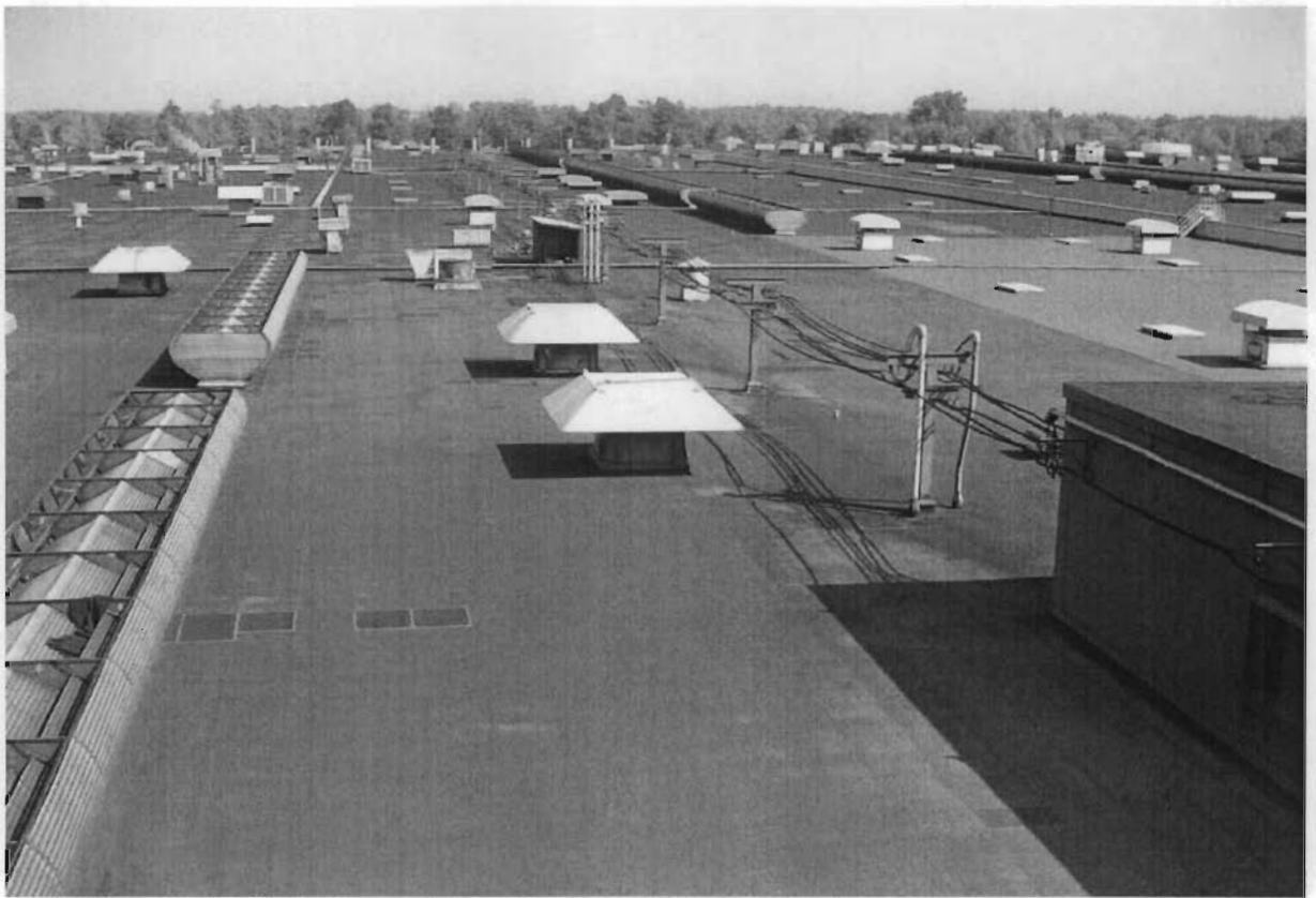
6. Facility roof after BMPs. Improved dust collection and daily roof cleaning.
