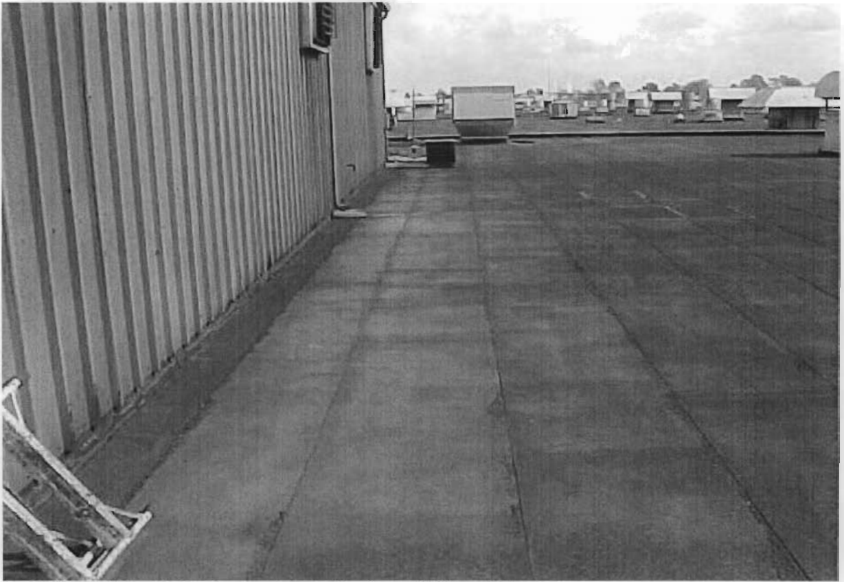
5. Facility roof after BMPs. Improved dust collection and daily roof cleaning.
